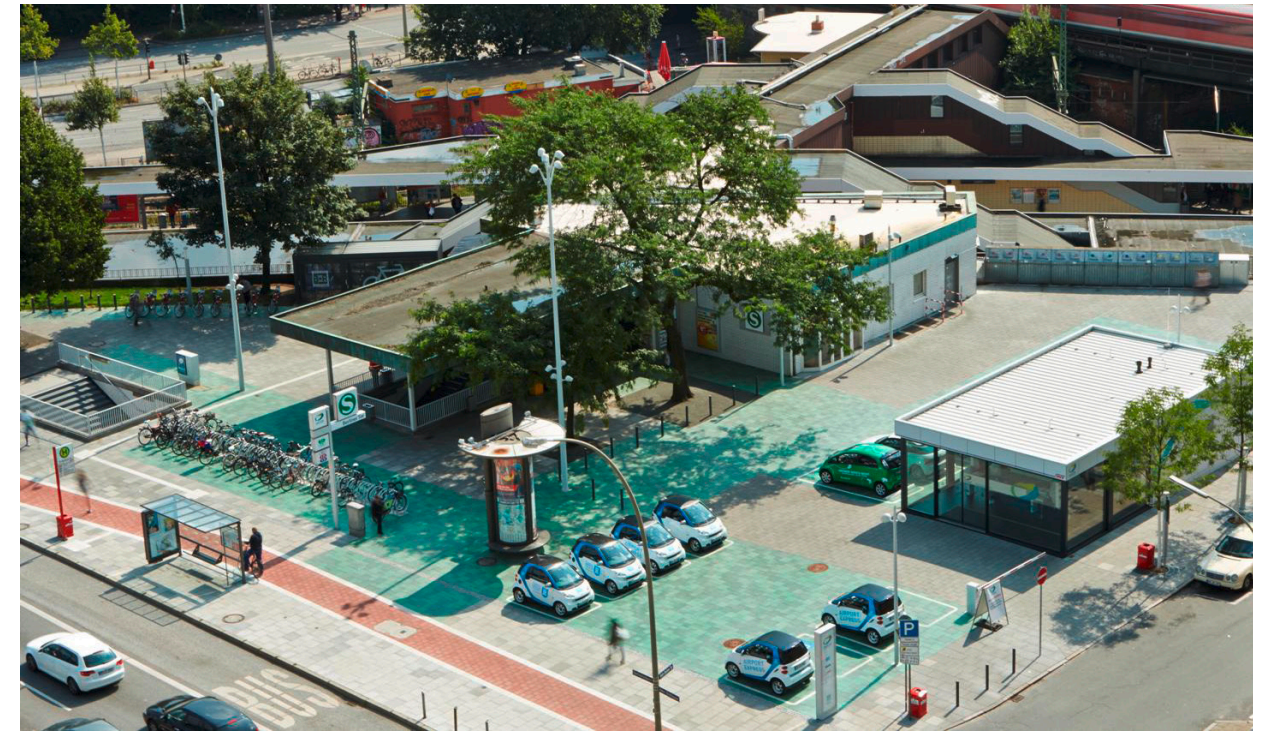
Berliner Tor Switchh mobility hub in Hamburg, Germany. Credit / Hamburger Hochbahn AG
